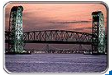
Marine Parkway Bridge
