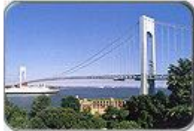
Verrazano - Narrows Bridge
