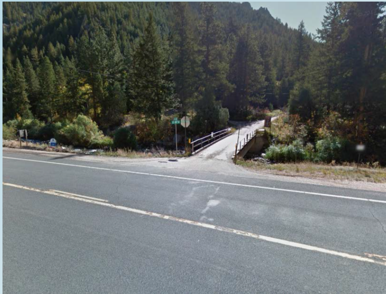
Local Access Bridge
