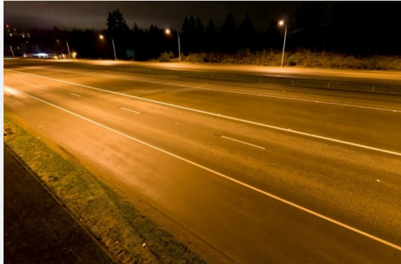
Before – HPS East View
