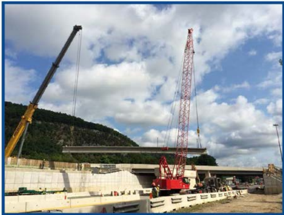
Setting concrete I-beams on the Interstate 84 eastbound bridge over Route 6, photo by John Pupa/PAIS.
